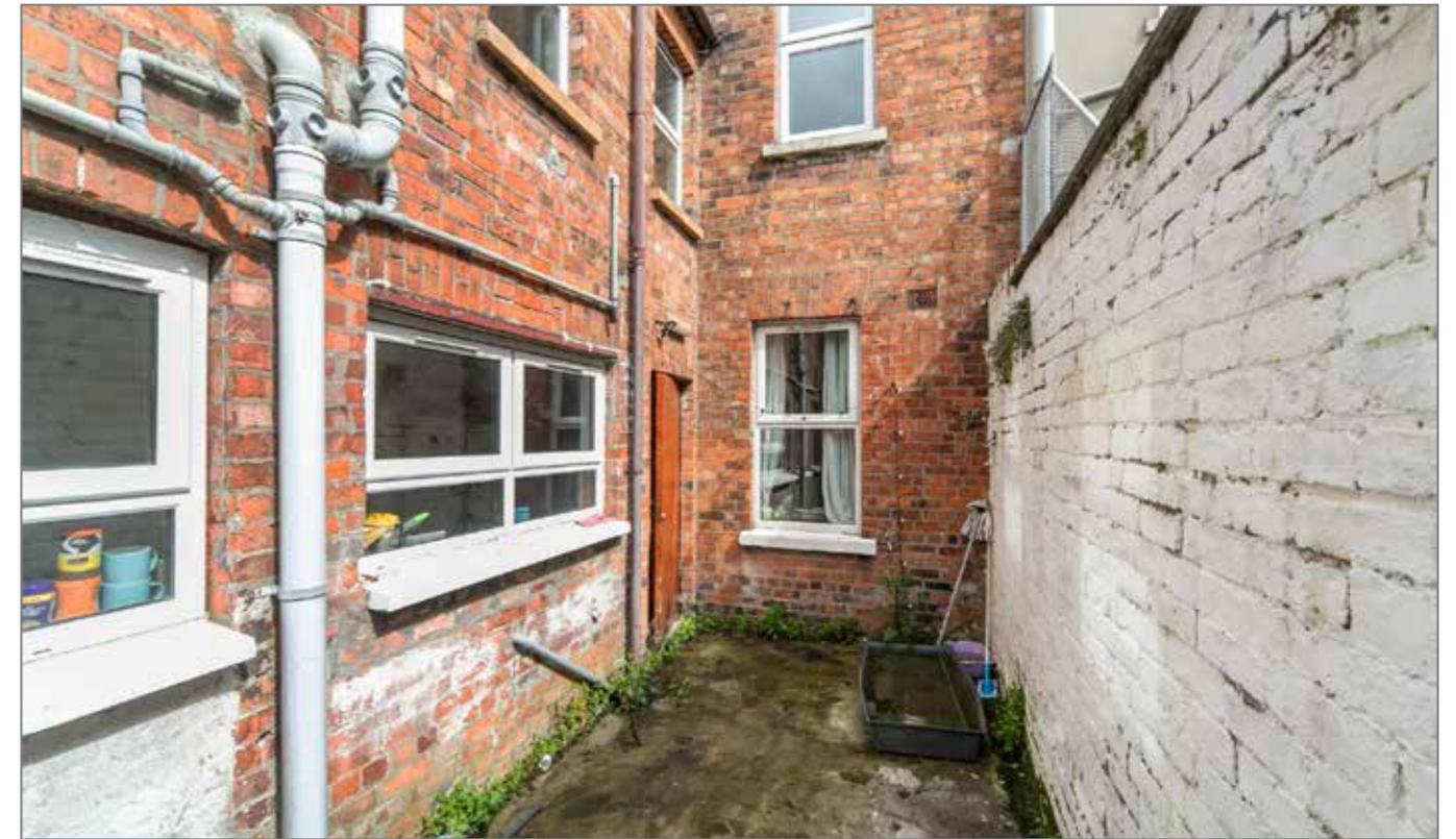
OUTSIDE Enclosed South facing private rear courtyard with hardwood access gate to bins
